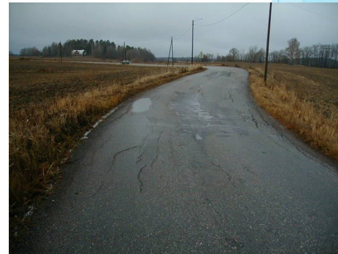
Frost actions & frost heave damage
