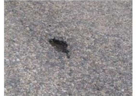
Hull Pothole
