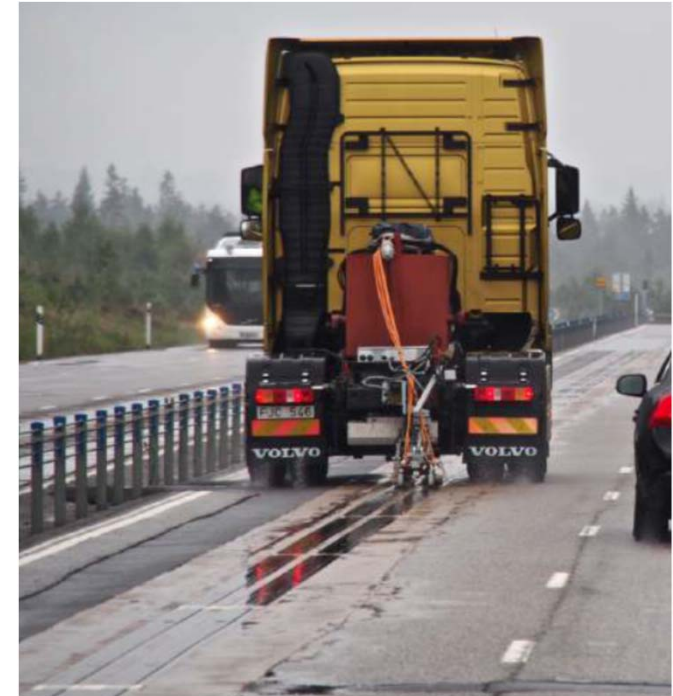
O. Olsson, "Project Report, Phase 1: Slide-in Electric Road System – Conductive project report," Viktoria Swedish ICT, April 2014
