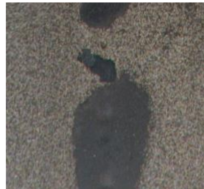
Reparert veg Patched road
